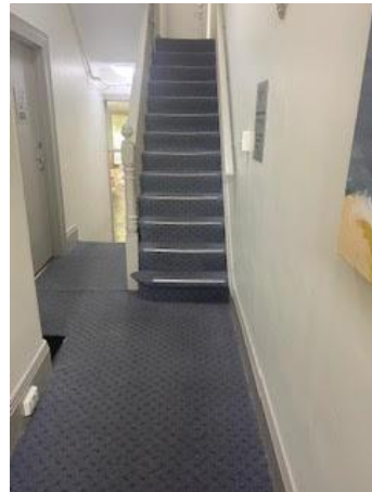
Fig 2: Existing Hallway carpet looking towards stairs form front door
