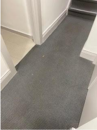
Fig 5: Existing WC entrance – carpet to be replaced by LVT planks
