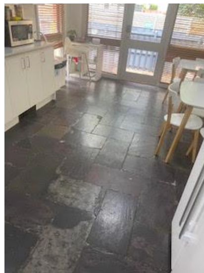
Fig 6: Existing slate floor in kitchen looking towards rear exit. Condition of substrate unknown at this stage – install entrance mat
