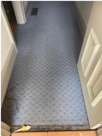
Fig 1: Existing carpet looking from front door to hallway
