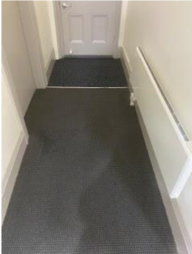
Fig 1: Existing hallway looking towards front door
