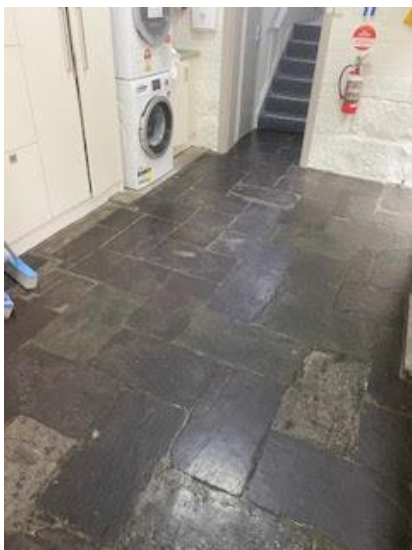
Fig 5: Existing slate floor in Kitchen area – showing concret plinth @ washer/dryer. Note concrete repair patches in floor.
