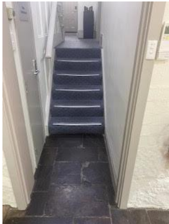
Fig 3: Existing lower hallway (slate) looking towards steps – replace with LVT planks
