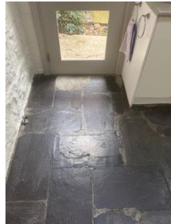
Fig 4: Existing slate floor in Kitchen looking towards RH Exit door – install entrance mat
