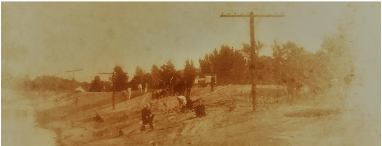
Construction of the highway through Mt. Vernon in about 1916.
