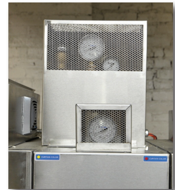
Stainless steel perforated boxes are used to protect the thermometers and gauges from damage.
