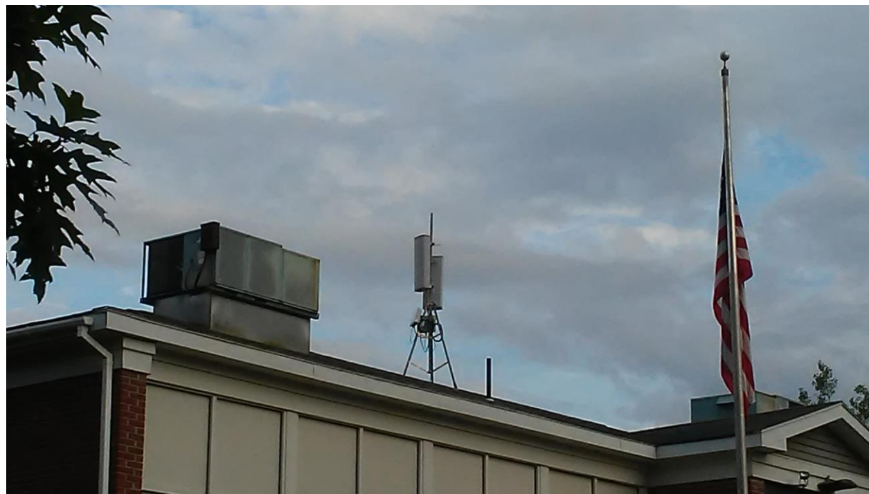
White Space Antenna on Roof of Millinocket Memorial Library
