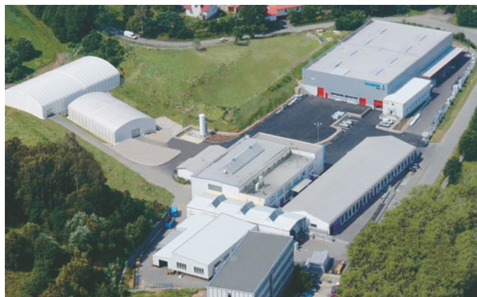
Plant Ledec nad Sázavou (CZ)
