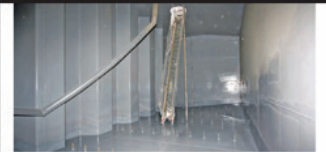
This image shows the heat curing of the MarineLine® tank coating system, developed by US-based Advanced Polymer Coatings as an alternative to building tanks of expensive stainless steel or having to employ restricted-use epoxy coatings in lining the tanks of chemical tankers.
